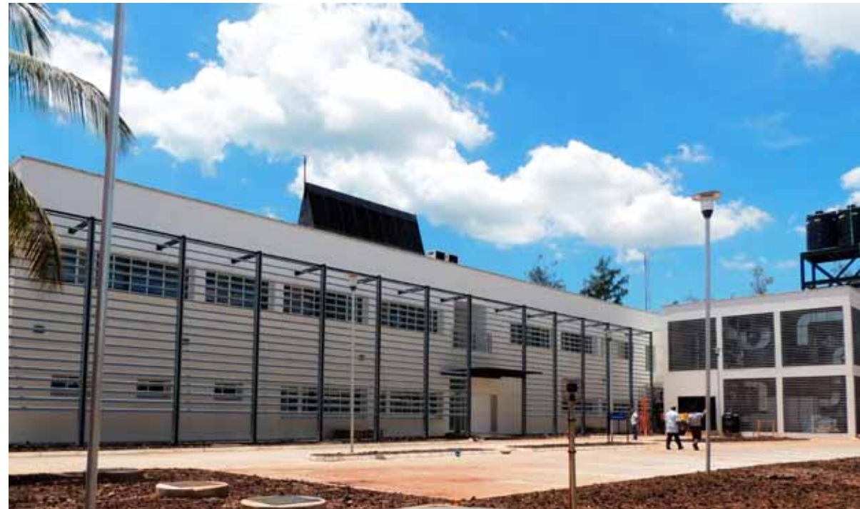
State-of-the-art Science Building, IITA, Dar es Salaam, Tanzania, April 2013. Photo by IITA
