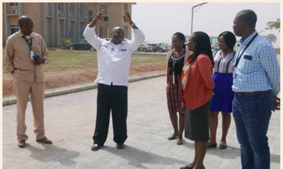
DG Sanginga (with raised arms) and staff at the Abuja Station on one of the newly constructed roads.
