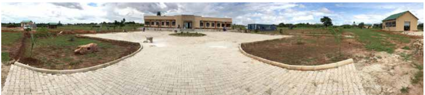
Panoramic view of the new structures. (From L-R: security gatehouse with drivers' lounge, generator house, main science and administration block housing staff offices, laboratory, small kitchen, and conference room, cassava processing building, and agricultural machinery fabrication building).
