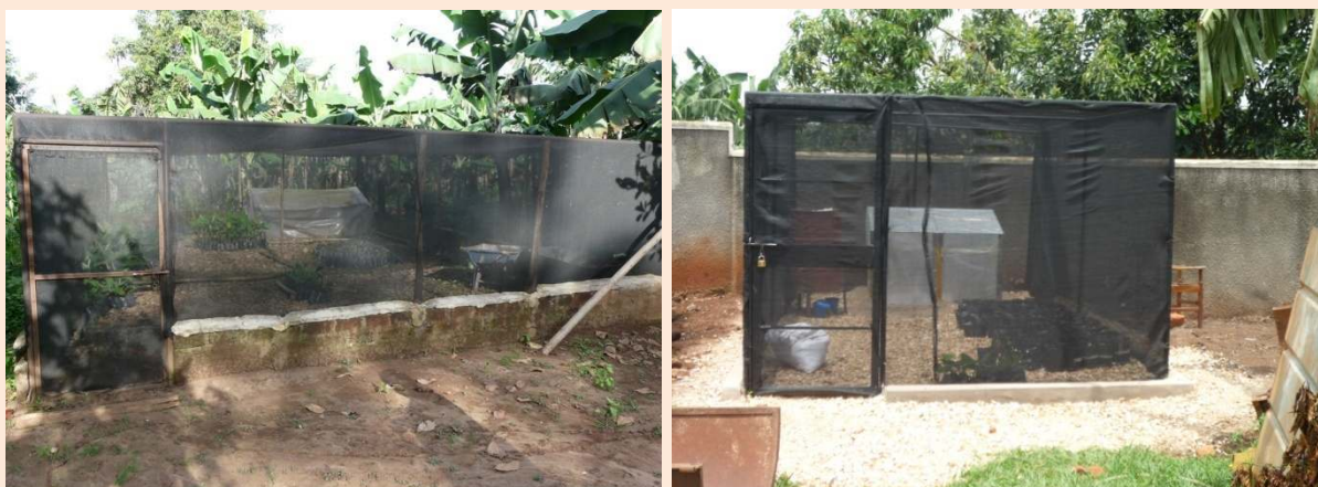
Fig. 5. A medium-cost shadehouse built with shadenets, metallic poles, cement and bricks.
