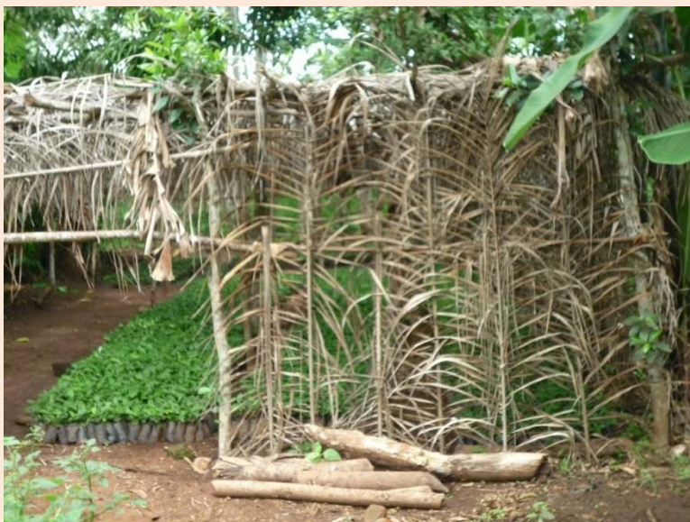
Fig. 4. Low-cost shadehouse built with timber and grass.
