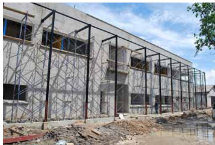
Work in progress on the IITA Science building in Dar
