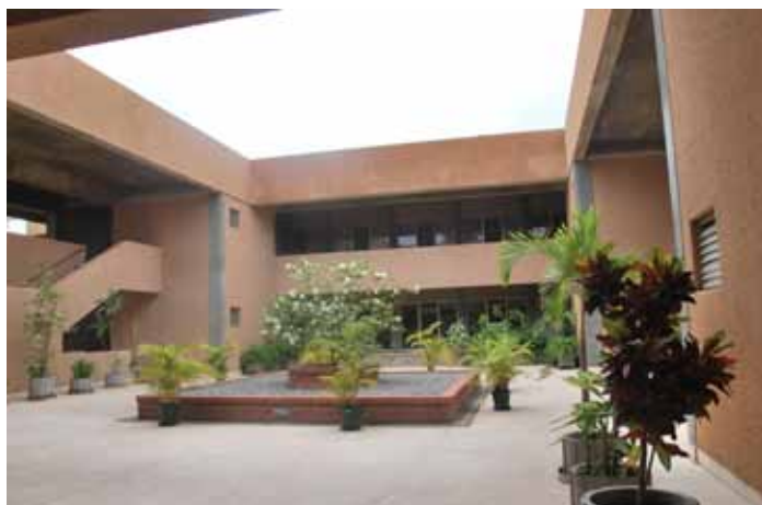
The newly painted Building 500 (FF Hill) in IITA Ibadan.
