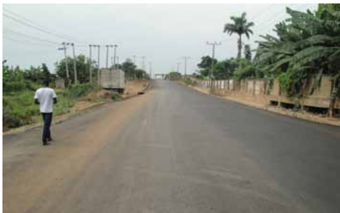
During his visit to the Oyo State Governor, Dr Sanginga made a request for the speedy construction of the by-pass road at Ajibode. The Governor responded and swiftly ordered the construction of the road.
