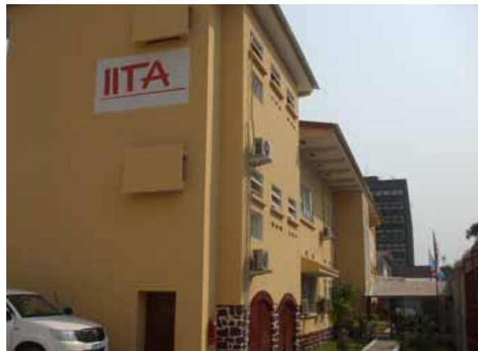
Recently commissioned IITA building in DRC.
