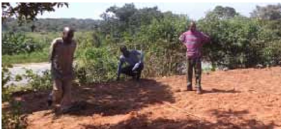
Engr Oluwatobi Oluwasola (second from left) leads in taking structural measurements and dimensions with extension officers and the site owner in Sanga, Nkhatabay.
