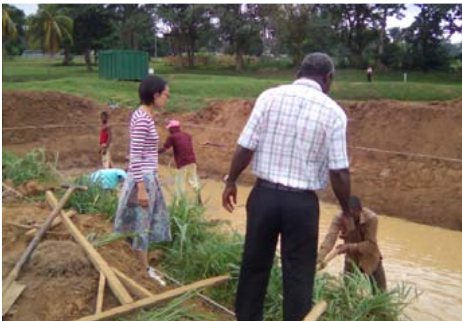
Ms Yukari supervising the construction of the ponds in Ibadan.
