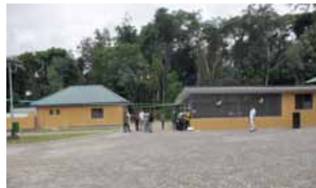
Side view of the new facilities
