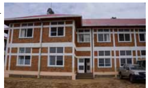
Part of the rehabilitated office buildings
