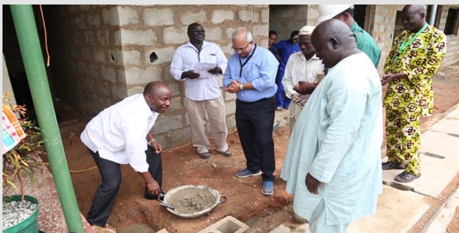
Dr Sanginga laying the foundation stone for the new laboratory.
