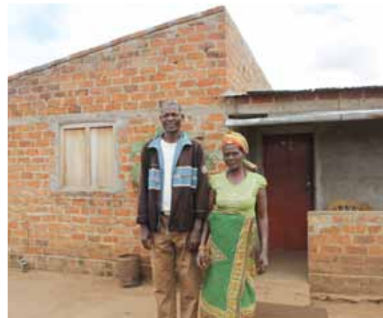
Mr Potocosse and wife in front of expanded house (right half is the old small house; left half are the newly added two bedrooms)
