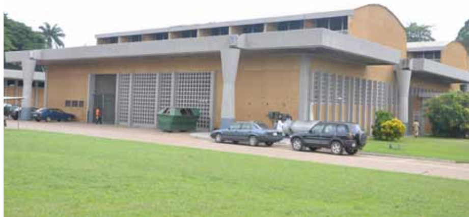
The new Threshing building
