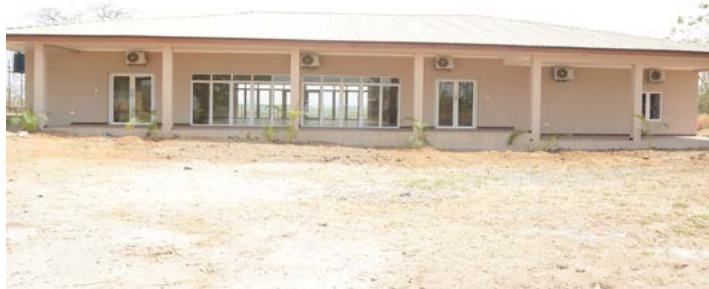
Newly constructed staff canteen.
