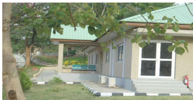
Reconstructed office building.
