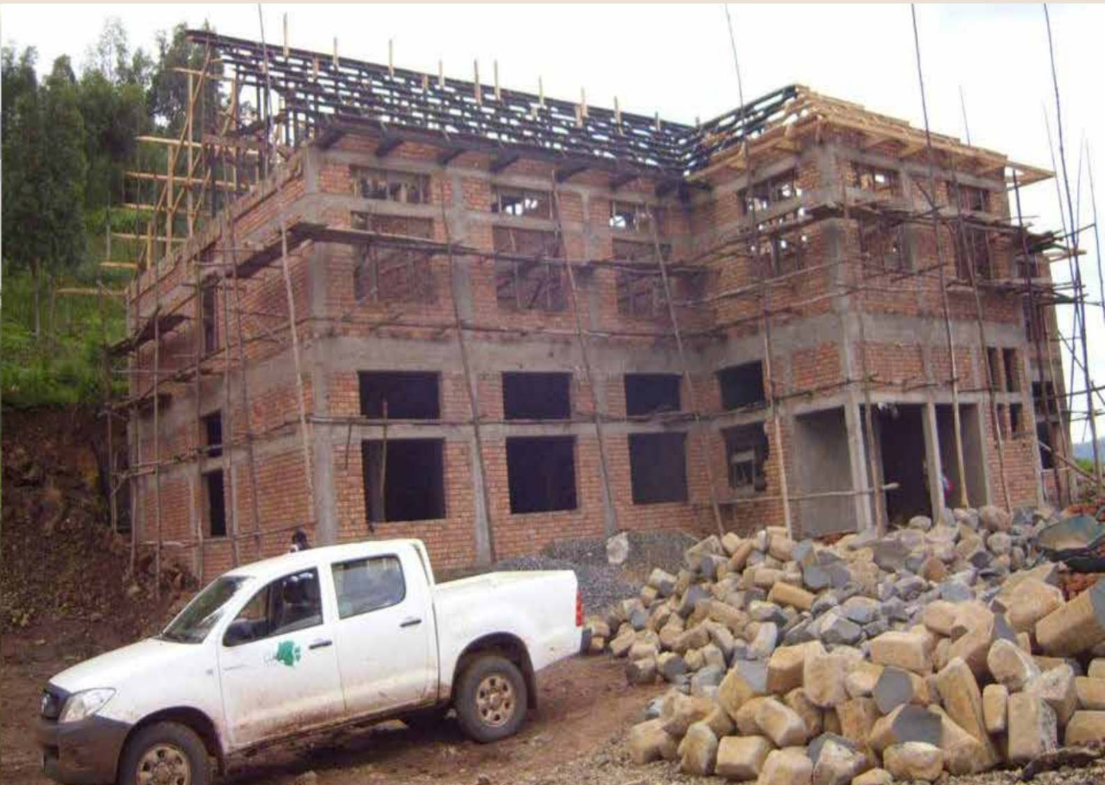
Construction of the first Building in 2009.
