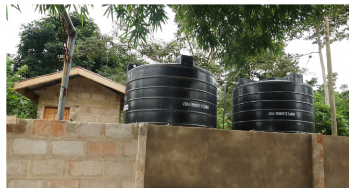
Irrigation system partly built (Photo Credit: IITA - Accra)
