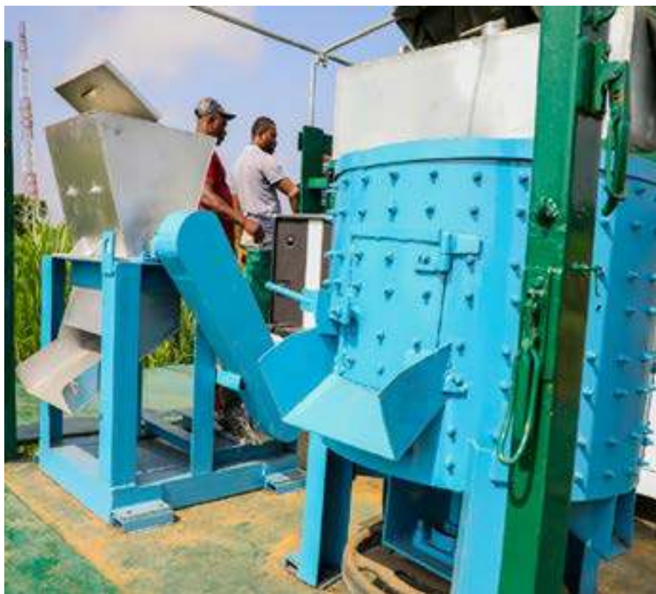
Installing a cassava processing unit.
