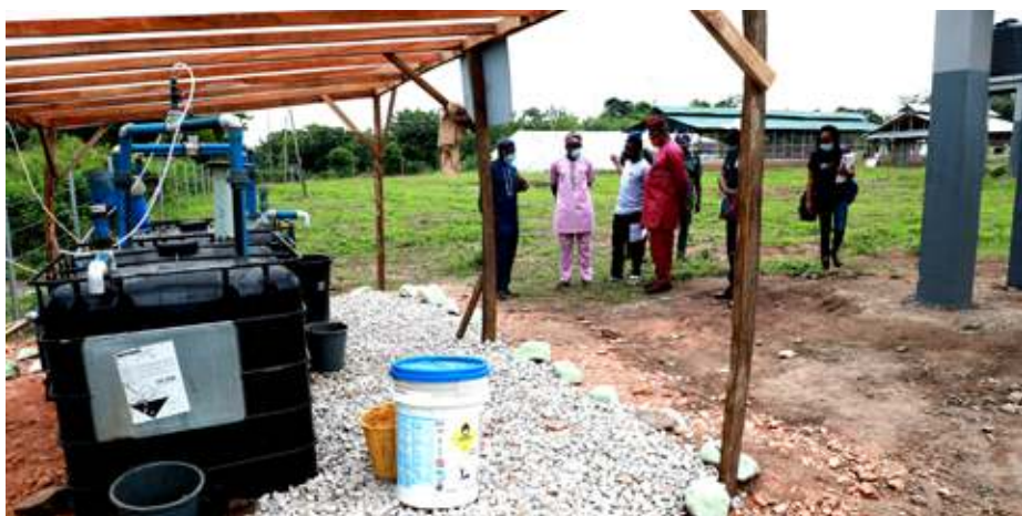
Top: The STEP center at Fasola school. Bottom: The biogas tank at Fasola school, converting waste to energy for the school and fertilizer for its farm.
