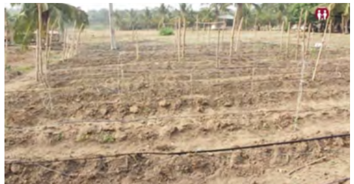
Open field after installation of the drip irrigation
