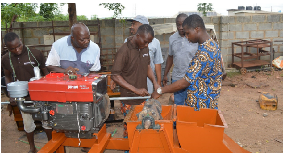
Fabricators constructing the wet hammer mill, supervised by IITA Postharvest Specialist Peter Kolawole (center background).
